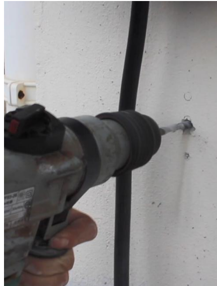
10. Use an electric drill to make holes in the drawing position
