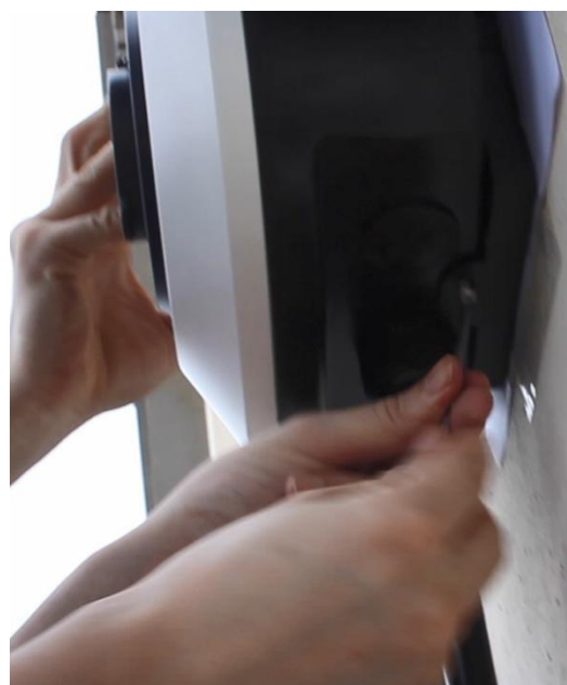
8.Tighten the anti-theft screw to ensure outdoor safety
