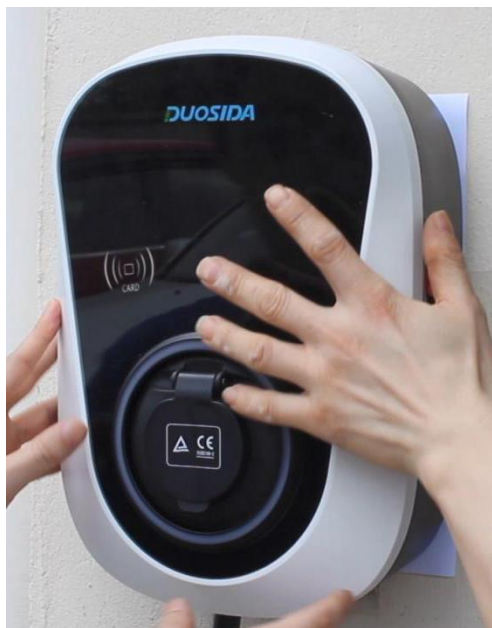
7.Hang the main body of the charging station on the mounting plate
